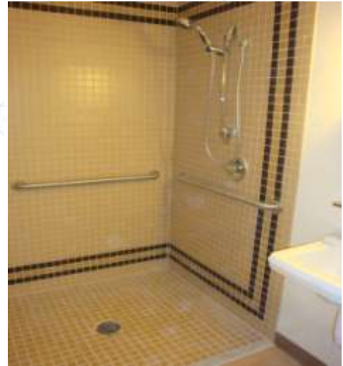
Shower Area After Renovation
