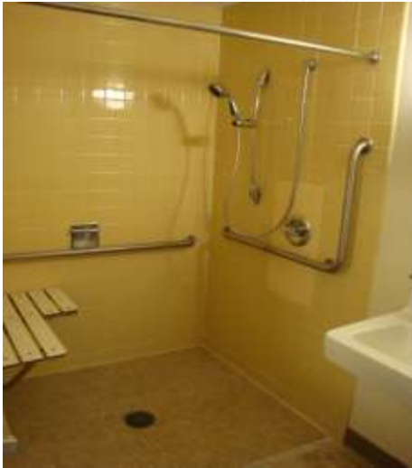
Shower Area Before Renovation
